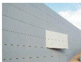
Kalesinterflex draws attention as a very light product not only among ceramic ware but tiles overall with its 12 kg/m<sup>2</sup> weight. Kalesinterflex, which offers suitable systems and detailed solutions to architects and project owners with its colors, texture, lightness and composite features like non-scattering when shattered, introduces distinction to spaces with its sizes ; 500x500 mm, 500x1000 mm, 500x1500 mm and 500x2000 mm, all derivatives of 500x3000 mm and its 15 special colors.
