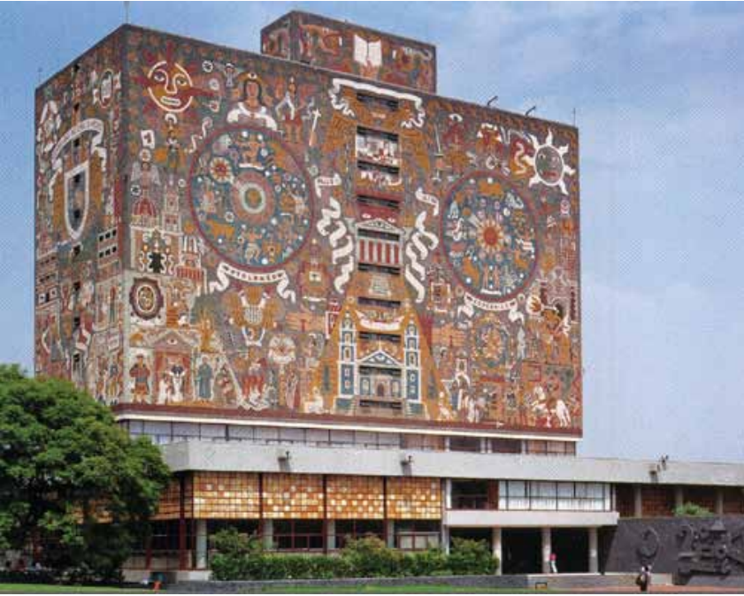
National University of Mexico, Central Library, Mexico City, 1953 (Architects: Juan O'Gorman, Gustavo Saavedra and Juan Martinez de Velasco)
