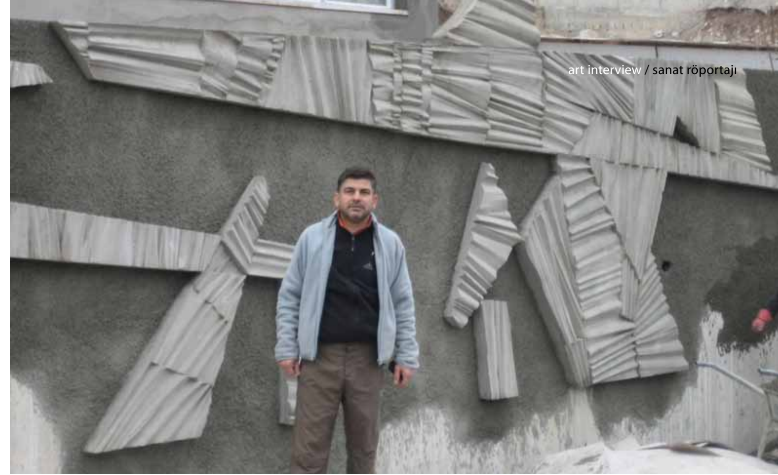
Ankara Sincan Heraeus Fabrikası giriş duvarı, 2008, beton, 15m/2.5m - Factory entrance wall, 2008, concrete, 15m/2.5m
